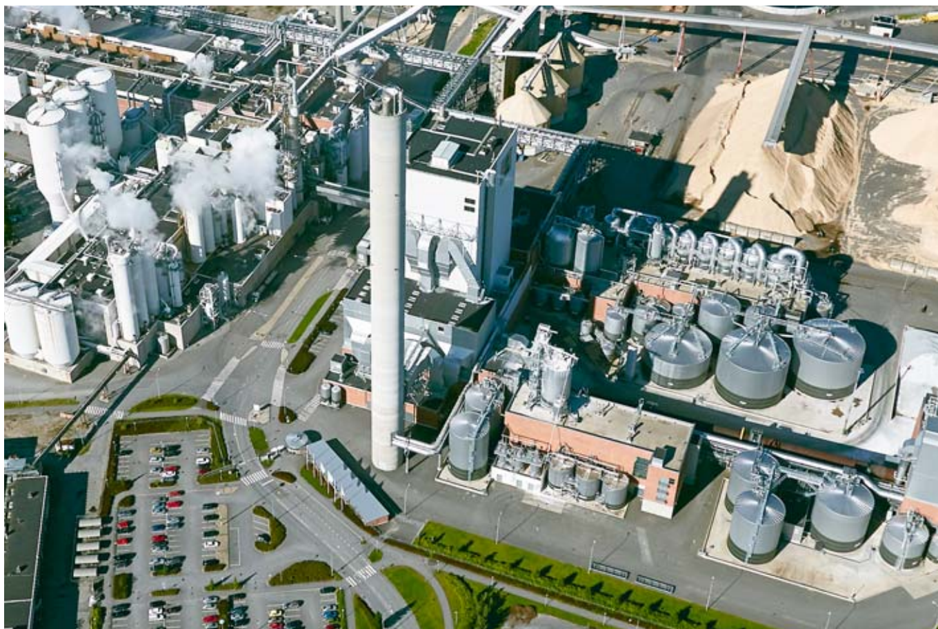
The pulp mill recovery island is one of the best recycling processes in industry. Chemicals for cooking are handled and used over and over again in pulp production.
